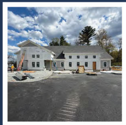
Ongoing Construction Ground Up Project
